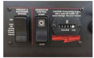
**TO STOP:** Turn OFF GENERATOR Selector switch on the 240v AC Panel. Allow the generator to run for a 3-5 minute cool-down period. Depress STOP momentarily on the lower part of the rocker switch. Turn OFF the GENERATOR BATTERY SWITCH over the 12v DC Panel.
