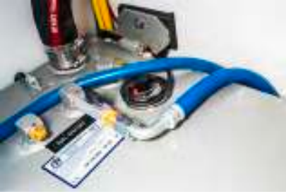
Starboard FUEL SHUT OFF
