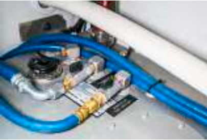
Port FUEL and GENERATOR FUEL SHUT OFF
