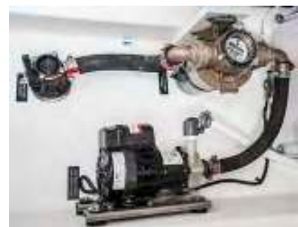
AC thru hull strainer and pump
