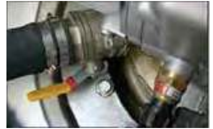
RAW WATER INTAKE VALVE open
