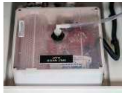
GRAY WATER SUMP
