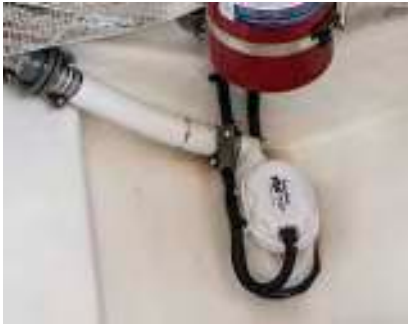
Aft BILGE PUMP
