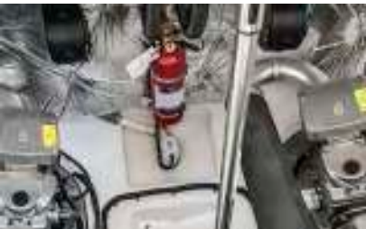
FIRE SUPPRESSION system and stern BILGE PUMP
