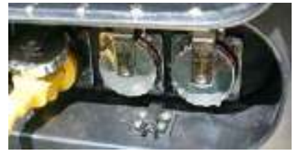
SHORE POWER INLET 1 is connected. None at SHORE POWER INLET 2. The receptacle on right is for Ethernet and coax TV connections.
