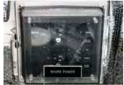
SHORE POWER BREAKER BOX
