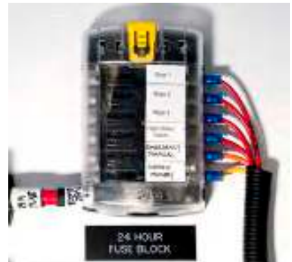
24-HOUR CIRCUITS connection terminal
